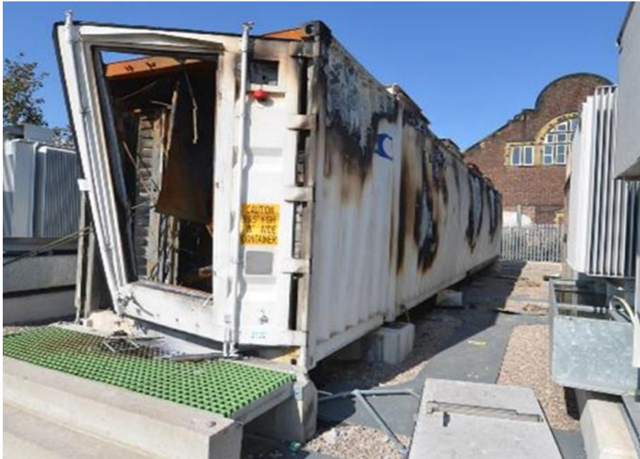
Figure 1: Carnegie Road Damaged Casing Exterior (Source: Merseyside Fire and Rescue Service)
