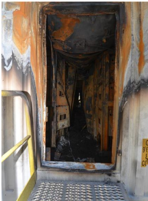
Figure 2: Carnegie Road Damaged Casing Interior (Source: Merseyside Fire and Rescue Service)
